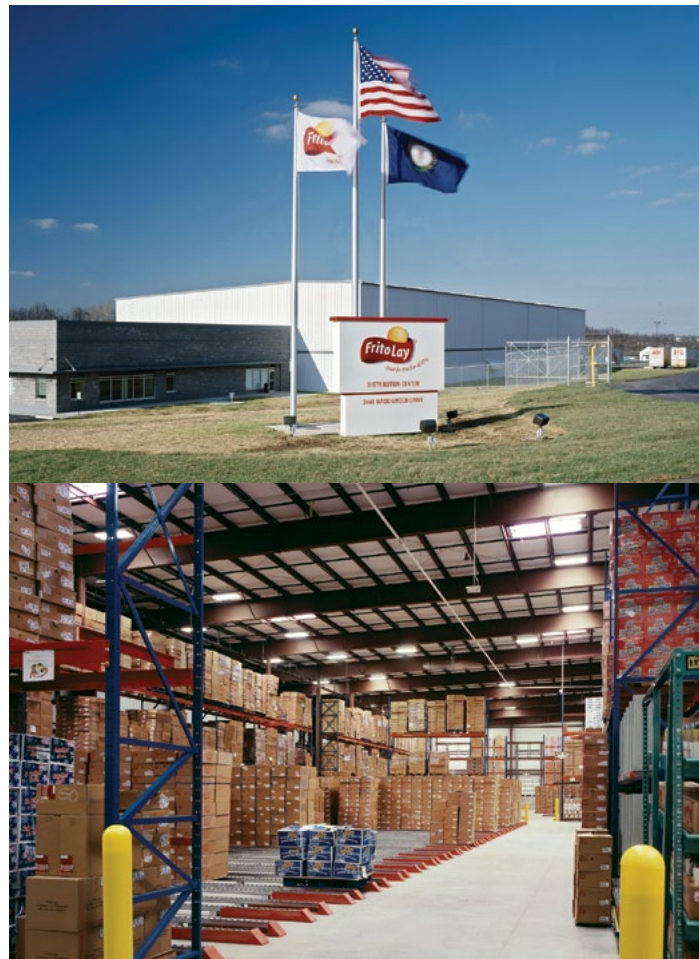
Frito-Lay Distribution Center (top and above), Lexington, KY
