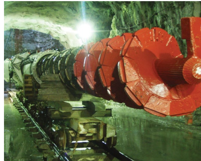
OSIS Augmentation Relief Sewer (OARS) Tunnel project, Columbus, OH
