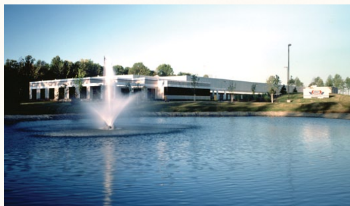
Kraft Foods facility, Twinsburg, Ohio
