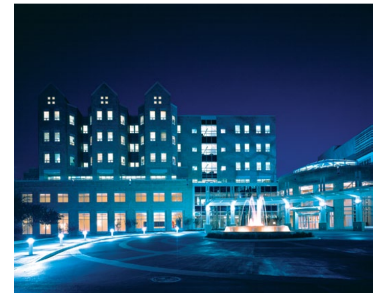
Baptist Children's Hospital, Jacksonville, Florida
