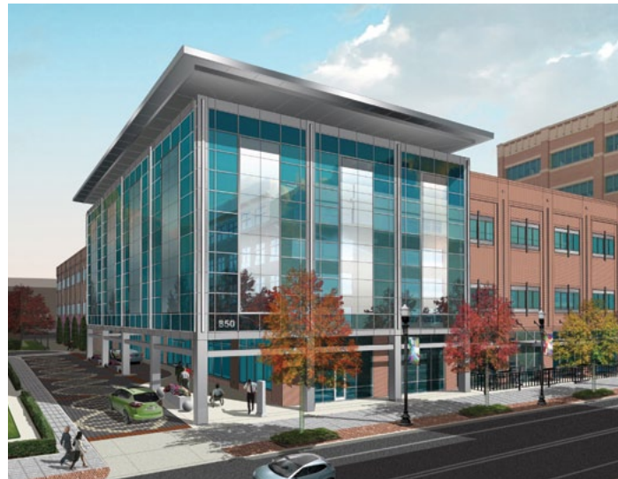
Maryland Proton Treatment Center rendering (above) and exterior and interior views of Scripps Proton Therapy Center, winner of ENR’s 2013 Best Projects Award of Merit, San Diego, CA (right)
