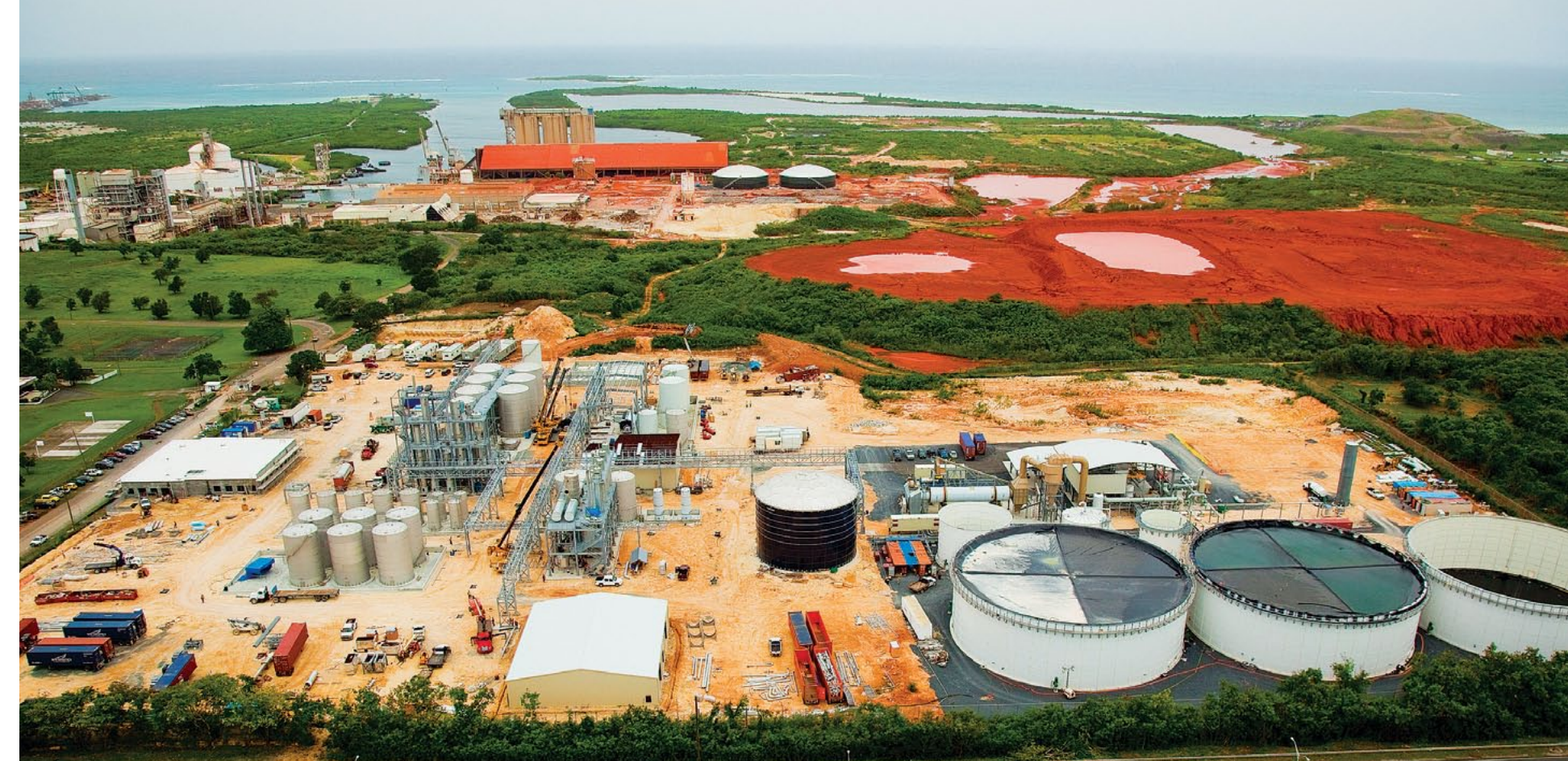
Diageo Captain Morgan Distillery WWTP St. Croix, U.S. Virgin Islands
