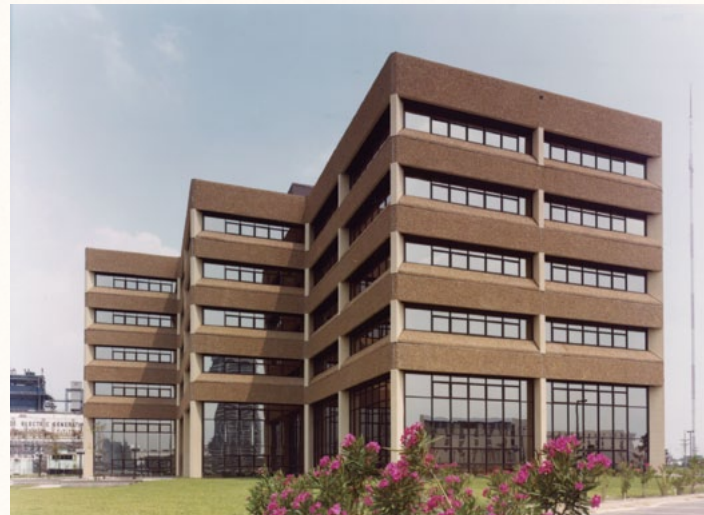
Duval County School Board Headquarters, 1981
