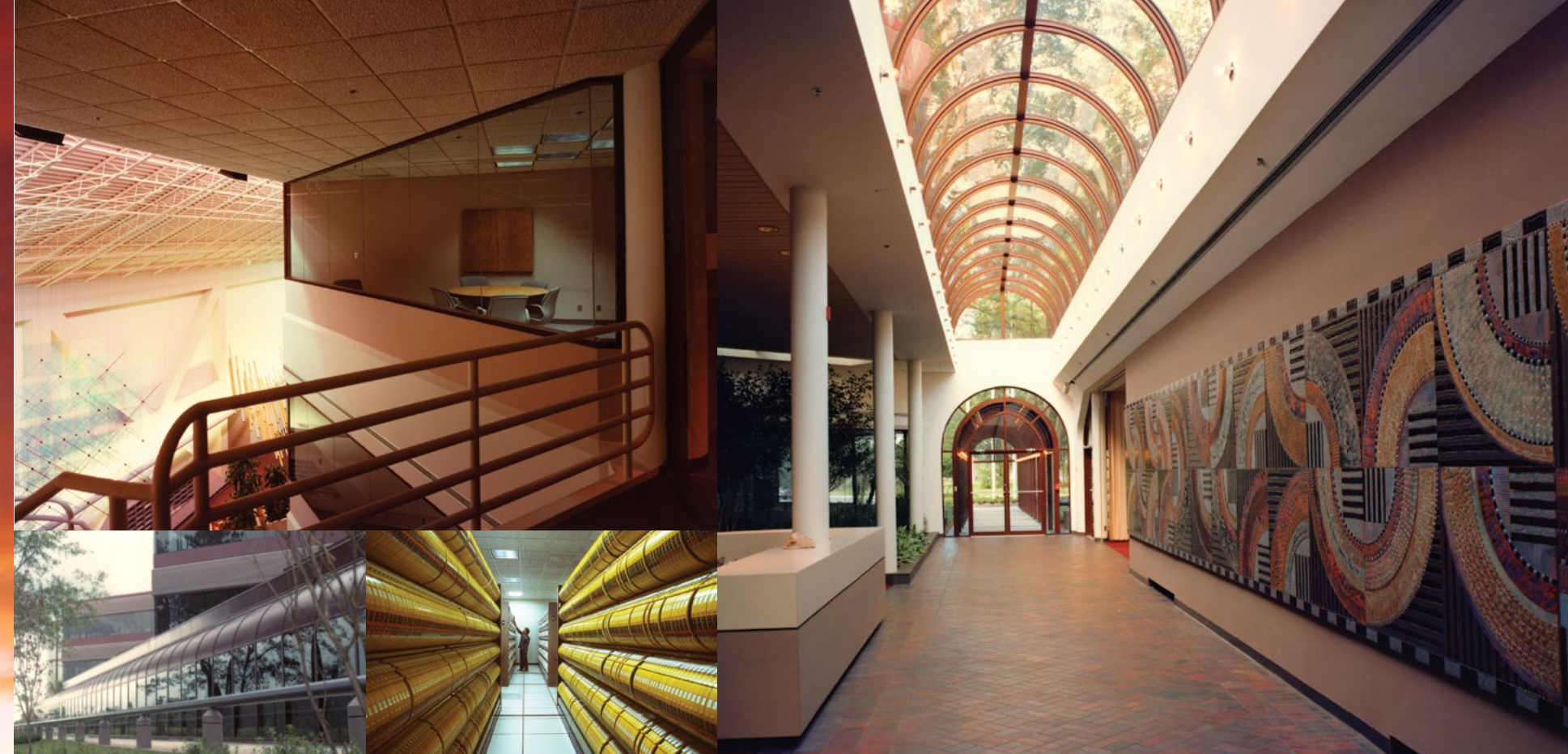
Exterior and interior views of the American Transtech Building (left and above)
